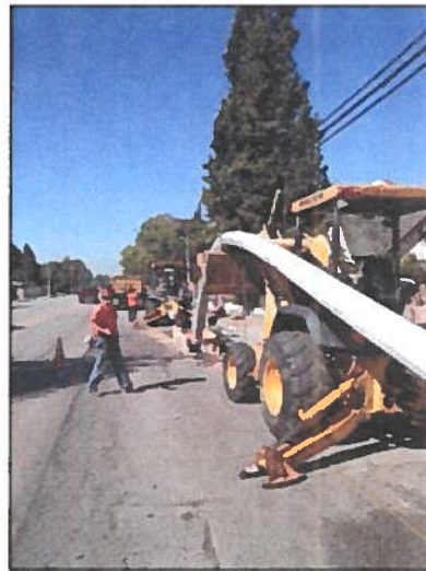
HDPE allowed the city of Covina to install a new pipeline without disruption important community areas like a hospital, baseball field, neighborhoods, and trailer park.
