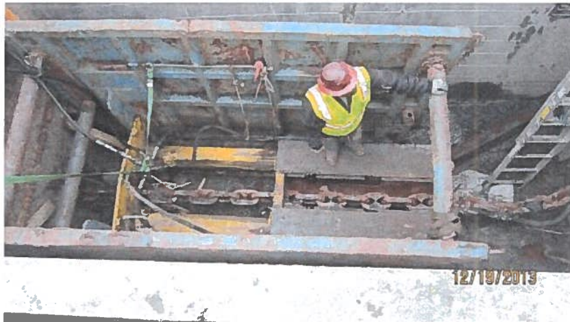
Static Bursting Machine
