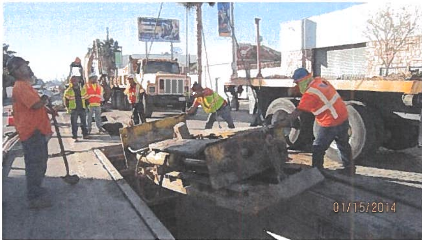
Static Bursting Machine being lowered into pit.
