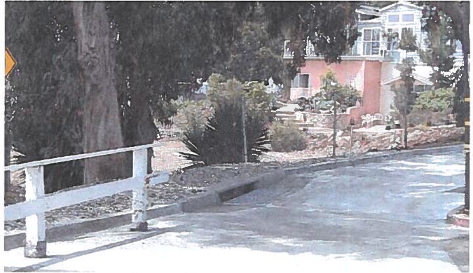
New catch basin with flowline remodeling.
